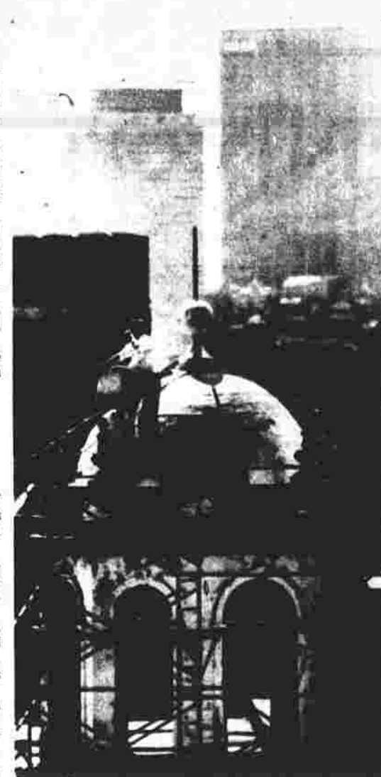
Gold leaf artist Jim McGurt takes a morning coffee break seated atop Harvard University's Adams House bell tower, 125-feet above the street. He has been applying three-by-three-inch squares of gold leaf to the dome of the dormitory since June 16. (UPI photo)
